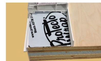
**Water Penetration Barrier** below each window and mullion with sill pan.
